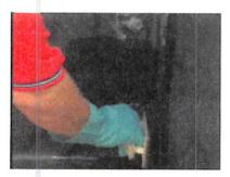
**Step 14-** Using a scrubber pad and holder; apply QuickPrime Plus Primer to both sides of the pig-ear shaped fold and beyond.
