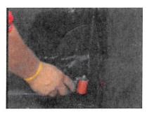
**Step 20-** Using a hand roller; roll the flashing to insure adhesion.
