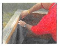
**Step 2**- Trim the PondGard panel so 4.0" (10.16 cm) will overlap the other wall to prevent leakage above the inside QuickSeam corner flashing.
