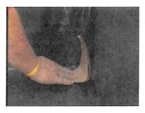
**Step 12**- Press the QuickSeam Corner Flashing tightly into the 90° angle and unfold into the corner.
