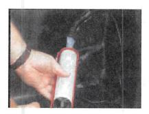
QuickScrubber™ Hand Roller **Step 21-** Apply a continuous bead of Lap Sealant HS or All Purpose Sealant over the edges of all tape or flashing.
