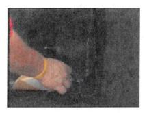
**Step 19**- Remove the release paper and center the tape or flashing in the corner and over the pig-ear fold.
