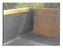
**Step 4**- Upon completion, the corner should look like this, with the PondGard panel slightly wrapped around the next wall.
