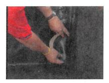
**Step 17-** Cover the pig-ear fold with a second QuickSeam Corner Flashing.
