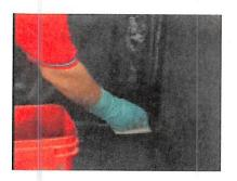
**Step 5**- Using a scrubber pad and holder; apply QuickPrime™ Plus Primer to a 14.0" by 14.0" (35.56 cm x 35.56 cm) area of the corner. Make sure to extend the primer past the adhered corner flashing.
