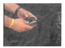
**Step 10**- Fold the corner flashing in half again to form a one quarter (1/4) circle.
