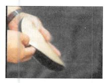
**Step 7**- Fold the corner flashing in half with the perforated edge on the bottom.
