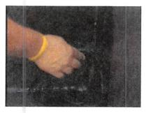
**Step 16-** Fold the pig-ear over using the primer as an adhesive to hold the fold of the flashing in place.
