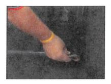
**Step 11-** Place the corner flashing 0.25" (0.64 cm) from the corner with the short side folded down.
